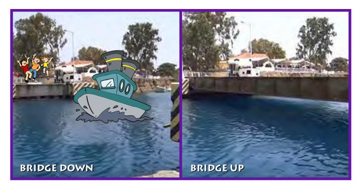
Wow! It's like nothing we've seen before. As a ship approaches the canal, this bridge sinks way below the water's surface. This allows the ship to sail "over" the bridge. After the ship passes, the bridge rises back up above the water so that the cars, buses and people can cross the bridge. That's pretty cool!
